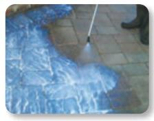
**STEP 1:** Flood coat sealer on surface with a low-pressure sprayer.
