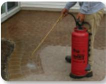
**STEP 1:** Spray sealer on surface with a low-pressure sprayer.
