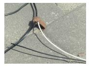
other half of the of the low voltage cable. You should have two connectors per light.
