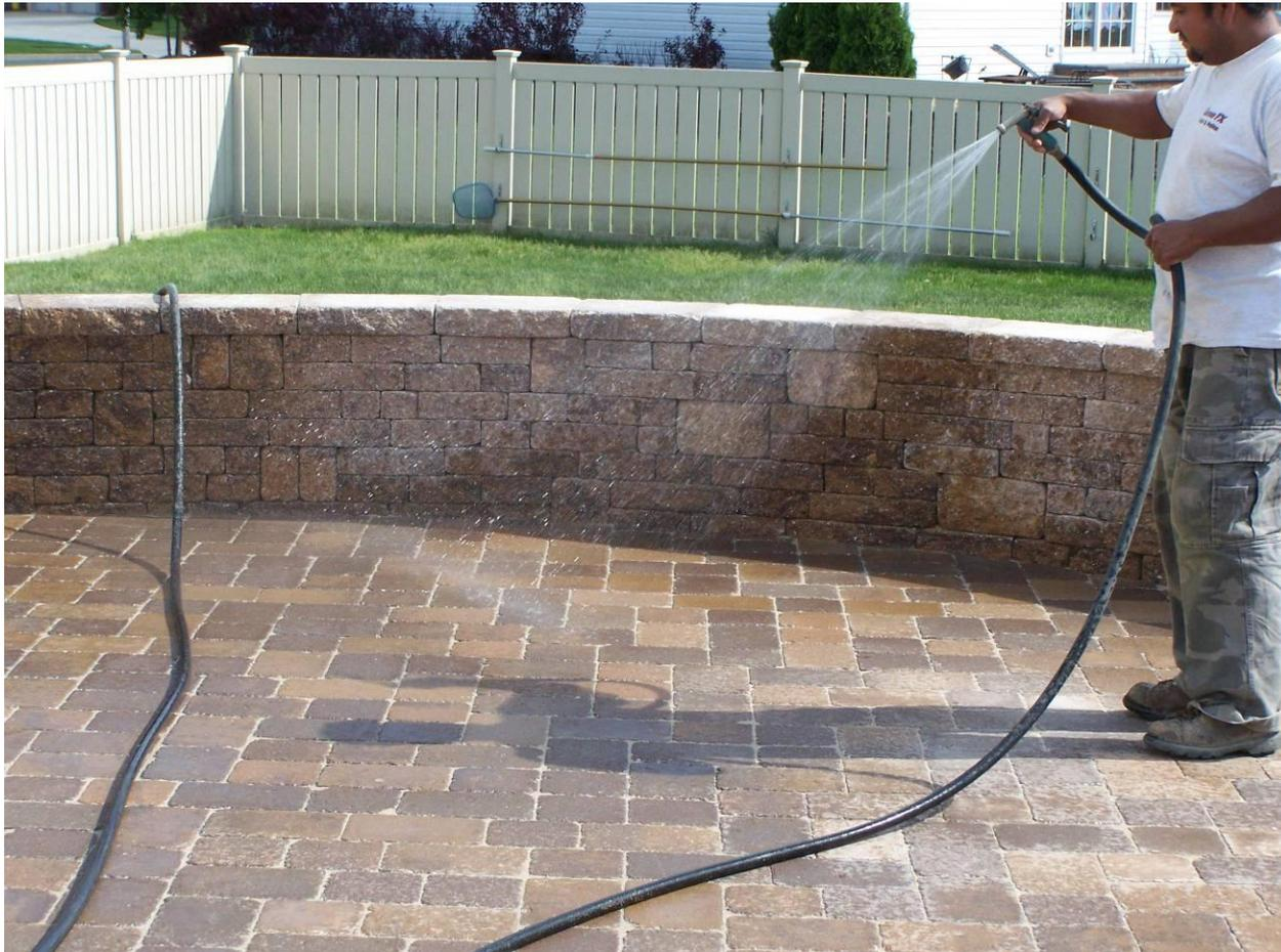
Check joints to make sure sands are wet to total depth of joint
