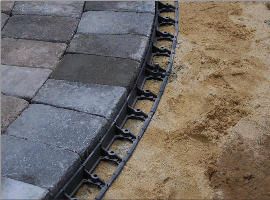
» Manufactured edge restraints like Snap Edge are designed by engineers and produced in controlled settings to provide consistent support. With a little training, anyone can install manufactured edge restraint correctly, quickly and easily.
