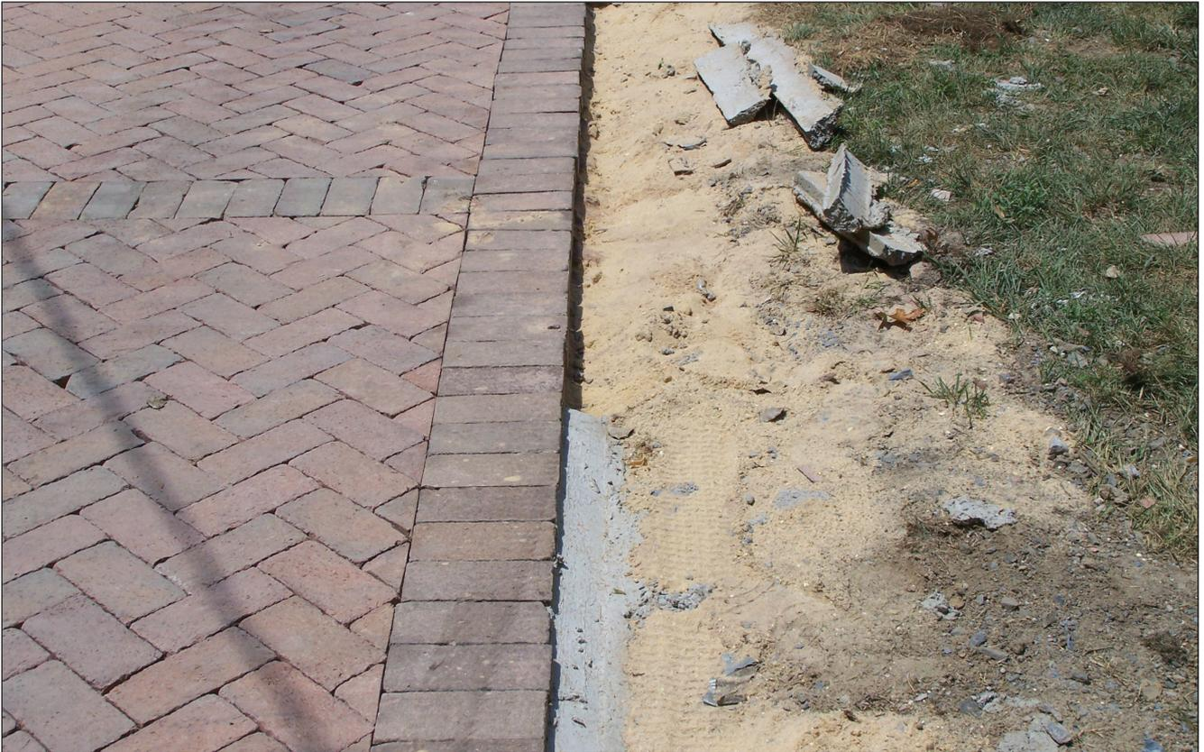
» Using concrete toe as edge restraint adds unnecessary risk to the success of a paver installation.
