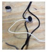
from the light fixture into the middle hole. Visually make certain all three wires are pushed to the back of the connector.
